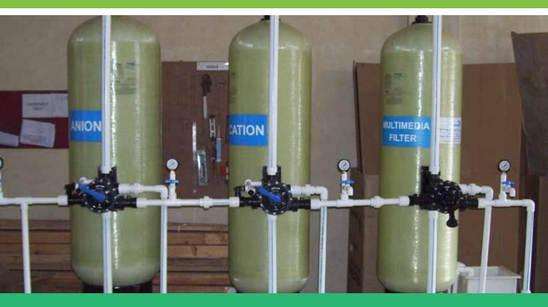
AGUAPURO FRP Water De-Mineralizers uses the proven Technique of Counter Current Regeneration; this involves the flow of raw water during Service, in opposite directions to each other. This ensures the consistent treated water quality which is always less than 2 ppm (TDS) or Electrical Conductivity less than 10 micro S/cm throughout the cycle.
